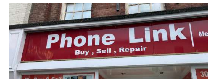
Poor example of low-quality, stuck-on plastic fascias with visible plastic fixings
