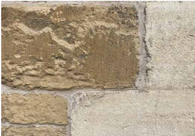
Yellow ironstone as part of local building
