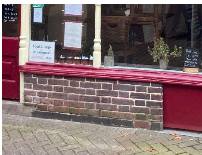
Stallriser in red brick features inset panels which enhances visual hierarchy to the façade design.
