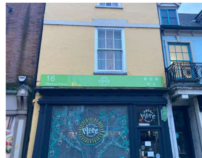
Poor example of a planted on fascia sign above the original fascia
