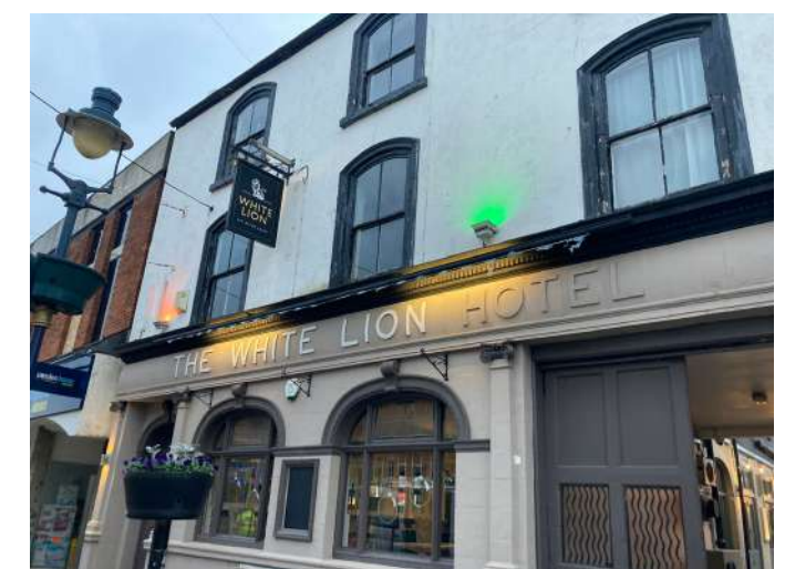
Inappropriate colour lighting on listed buildings
