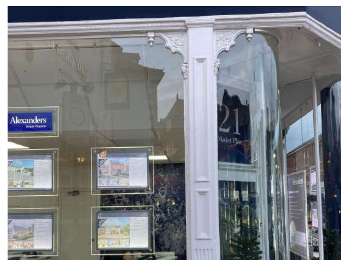
Traditional shop window and mullion featured intricate carvings retained in the existing shopfront
