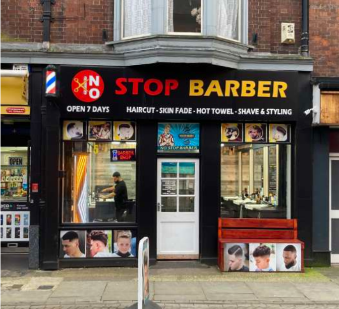
Poor example of neglecting the fascias and cornices in design, the oversized board obscures original architectural details
